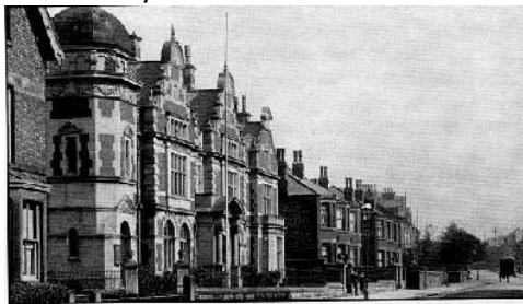
Manor Road Police Station, Liscard, opened 1900
