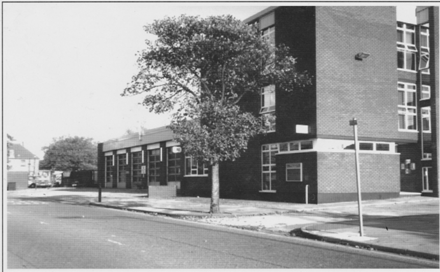
Mill Lane Fire Station, Wallasey, opened 27 March 1974
