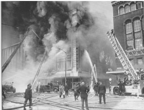
Henderson's store fire Church Street, Liverpool 22 June 1960
