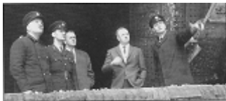
Frank Uriel points out the damage to officials attending the New, Brighton Tower
